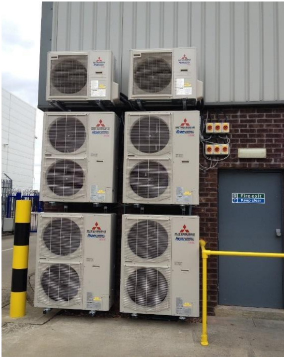
6 Air Conditioning Units – Supplied & Installed
