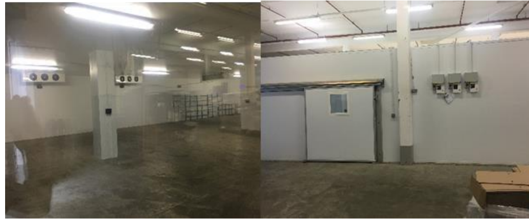
45ft x 40ft Cold Room – Supplied & Installed
